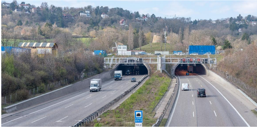
A81 Engelberg tunnel Leonberg
