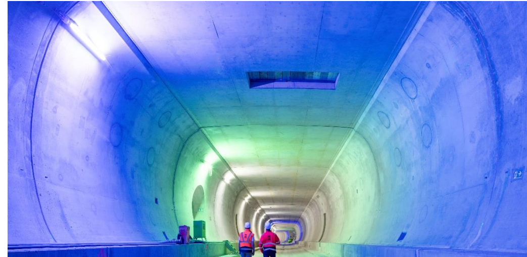
Rosensteintunnel in Stuttgart Bad Cannstatt
